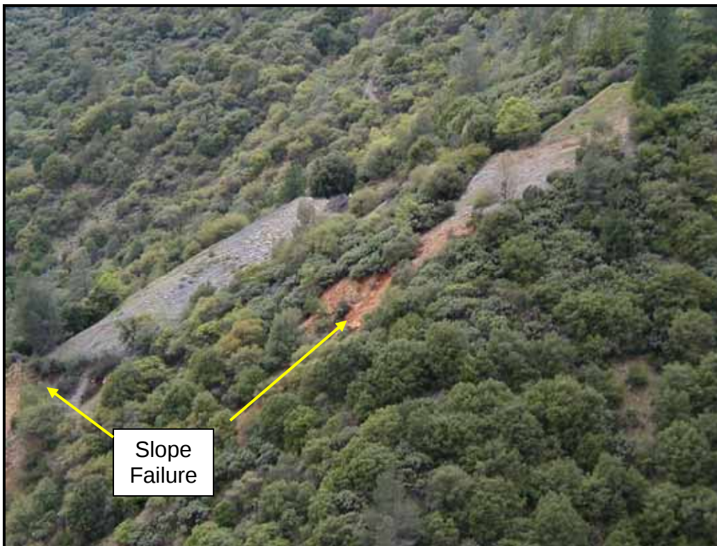
Photo 2. Slope Failures Waste Dumps #2 and #4.
